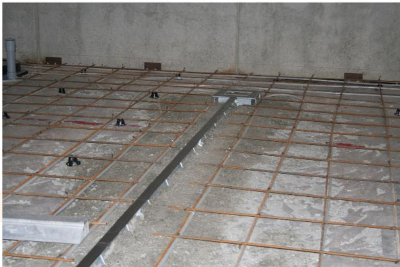
6. Once the concrete slab is firm, remove the tape from the slot and clean out the U-drain and sump pit using the Paddle.
