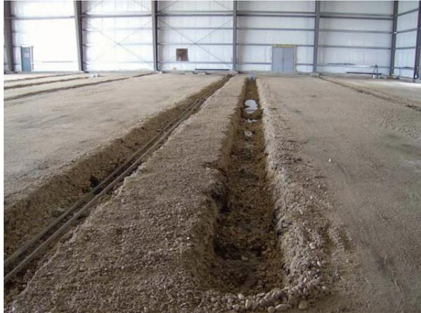
2. It is recommended to pre-pour a concrete pad underneath the sump pit to it can be properly secured. If no pad is poured, peg the sump pit down before the U-Drain is connected.
