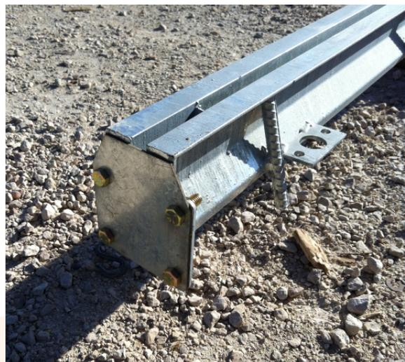
4. Fasten the E-Z Mount Brackets at each U-drain bracket interval, using the hardware supplied. Pound appropriate lengths of rebar into your base material with the rebar running through the conduit portion of the E-Z Mount Bracket. Make sure that the tops of all sections are level. When the correct levels are achieved, tighten the set bolts on the E-Z Mount Brackets to secure the U-Drain.
