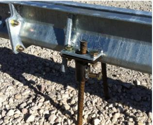
5. Once the U-drain is secured to the E-Z Mount Brackets and the appropriate floor height is found, tie rebar from the floor grid into the rebar on the U-drain assembly, for structural support. Cover the slot opening with duct tape.
