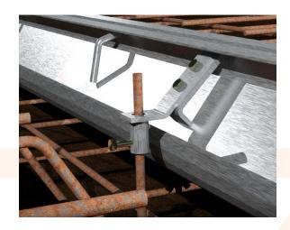
7. Once the U-drain is secured to the E-Z Mount Brackets and the appropriate floor height is found, tie rebar from the floor grid into the rebar on the U-drain assembly, for structural support. Cover the slot opening with duct tape.
