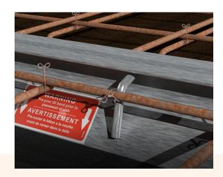
8. To guarantee that the U-drain will not float, it is recommended that the concrete be poured in two stages. First, pour the concrete till the warning sticker on the U-drain assembly and let the concrete sit. Once adequate time for the concrete to set has elapsed, complete the floor slab. The use of a pencil vibrator is strongly recommended to make sure that the concrete has completely surrounded the U-drain leaving no bubbles or voids.
